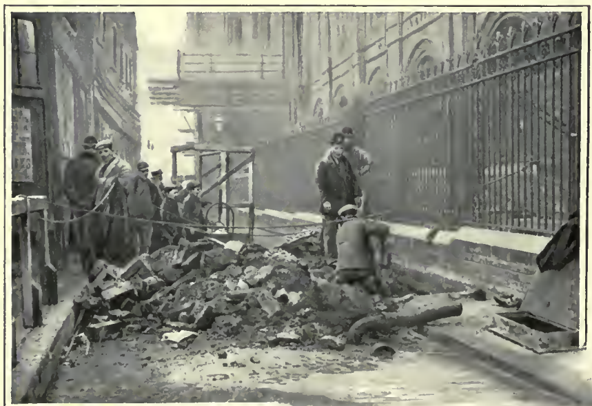
REPAIRING A BURST WATERPIPE.
