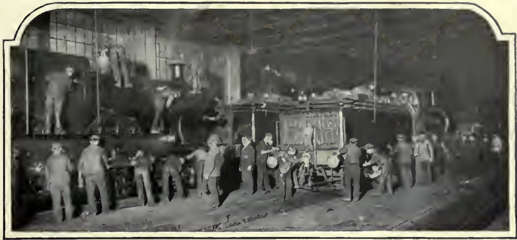
CLEANING ENGINES (WESTBOURNE PARK).
