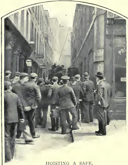
HOISTING A SAFE.
