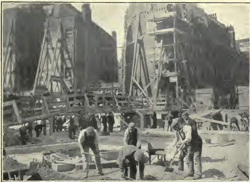
A TEMPORARY BRIDGE.
