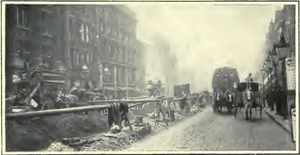
WORKING IN TRENCHES.
