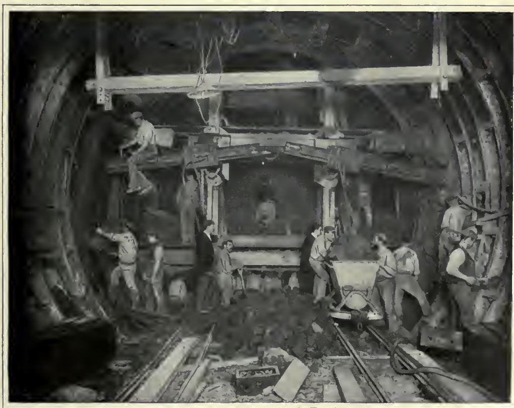
EXCAVATING A TUBE RAILWAY: AT WORK IN THE "SHIELD."
