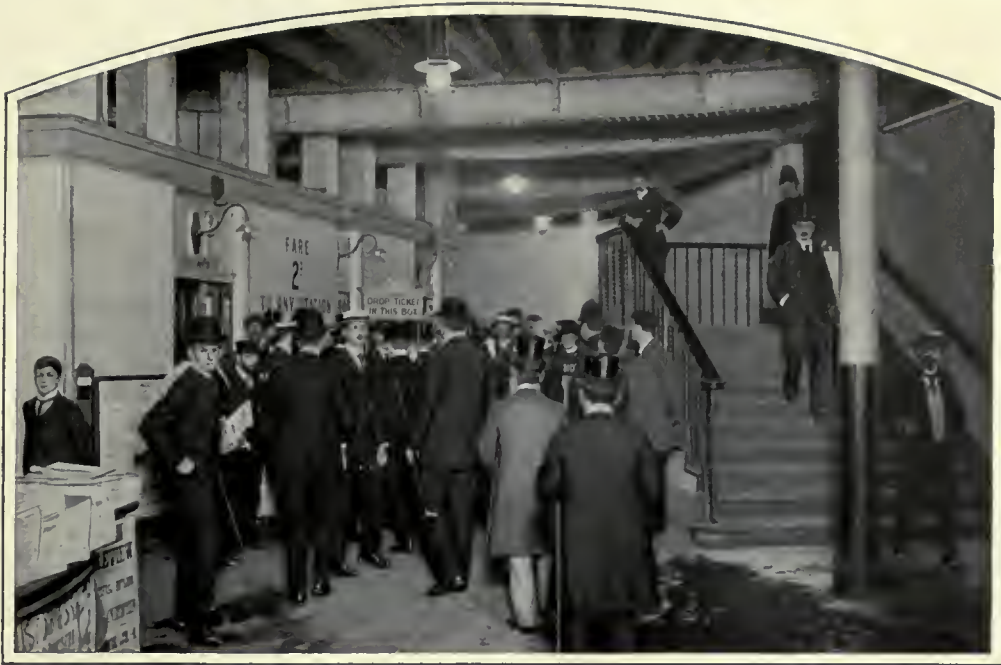
WAITING FOR THE LIFTS AT THE BANK STATION (CENTRAL LONDON RAILWAY).
