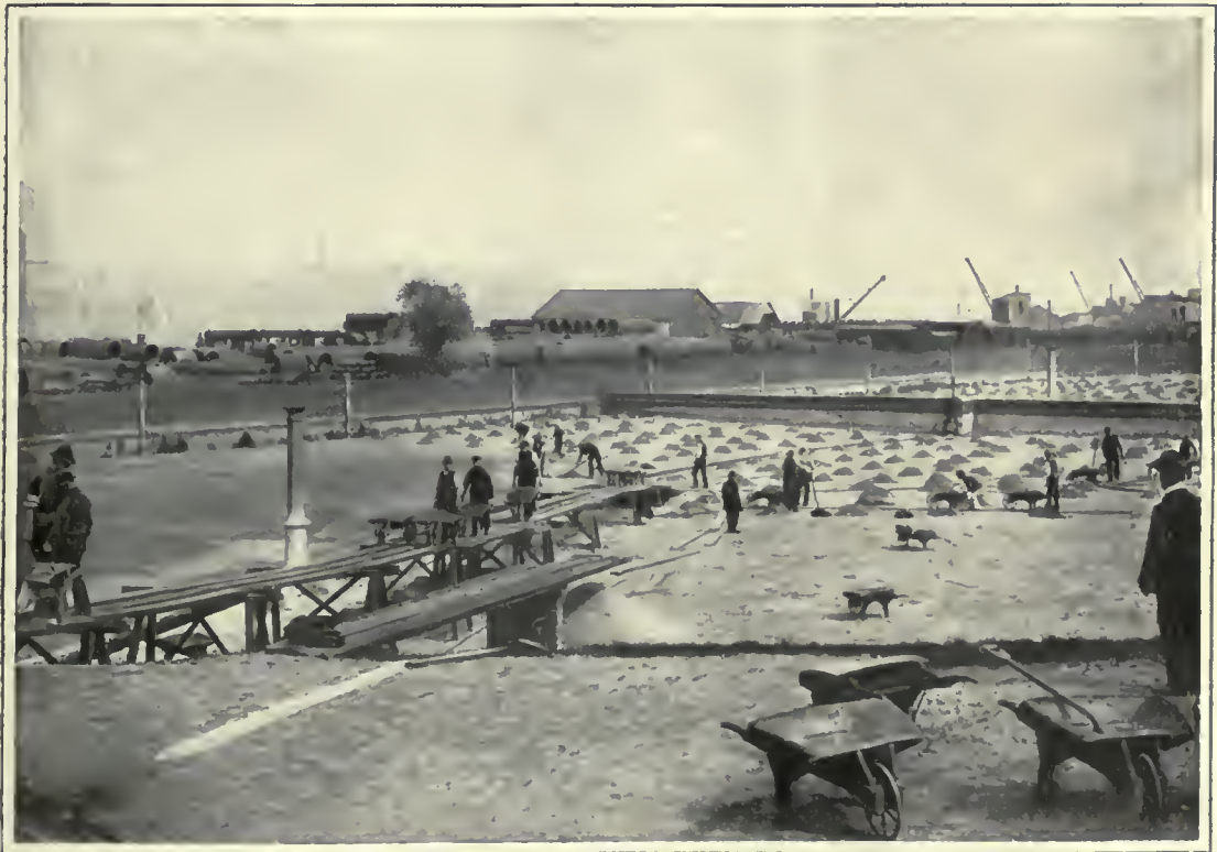
CLEANING A FILTER BED (BATTERSEA).
