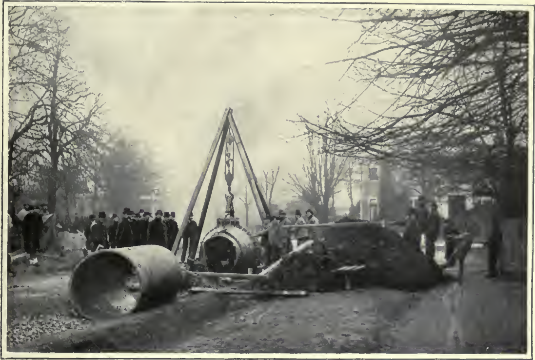
LAYING A BIG WATER MAIN.
