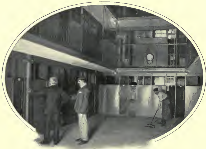
L.C.C. LODGING-HOUSE (PARKER STREET) : CUBICLES.
