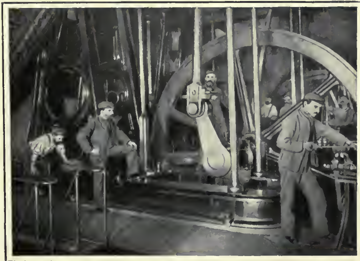
PUMPING ROOM (BRIXTON HILL WATERWORKS).
